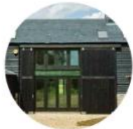
Sliding 'Barn' Doors
